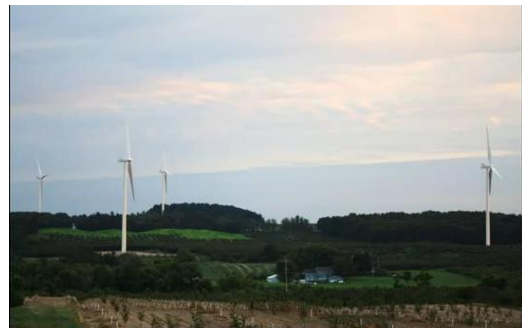
The Lake Winds Energy Plant surrounds homes in Mason County.
